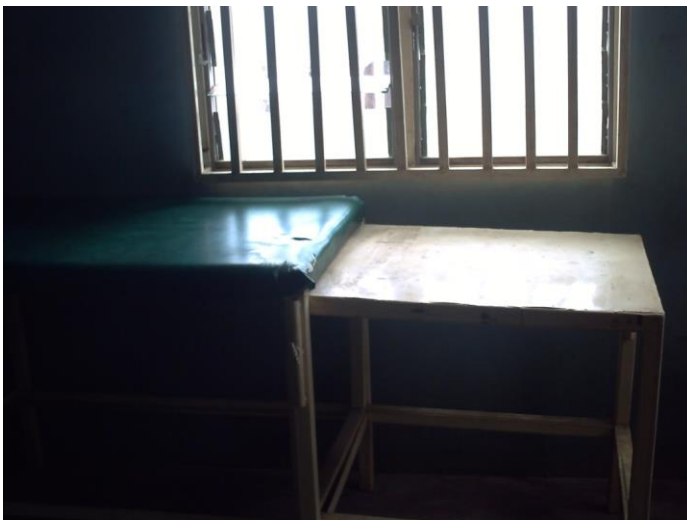
D: Sample of delivery beds with rusted metal part in the maternity centre
