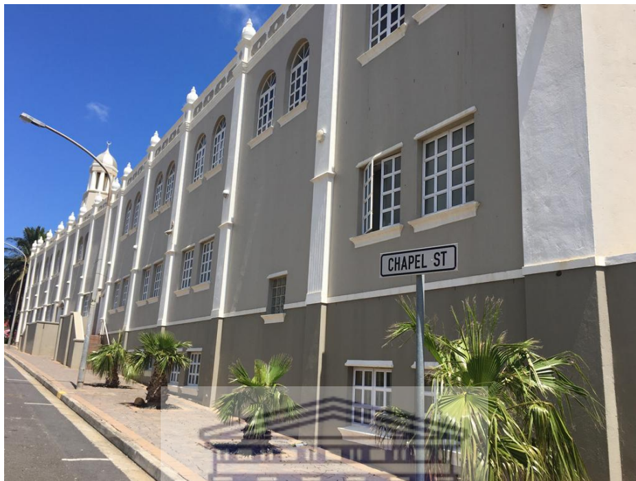
Figure 4: The Zeenatul Islam Mosque, one of the long-standing mosques in District Six (Source: Author)
