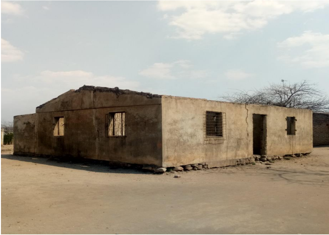
Figure 5: An abandoned house in Bagamoyo. September 2018.
