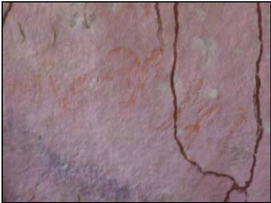
III. 31. Natural Hazard: Insect tunnels mastic on pictograph (Photograph taken by writer, 2002 December)
