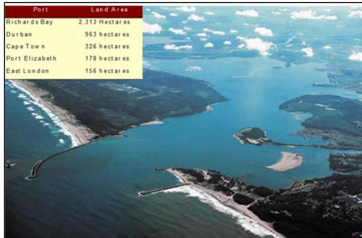
Figure 3.3: Richards Bay Port (extracted from Transnet Port Terminals, 2013)
