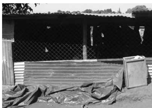
Rudimentary broiler house
