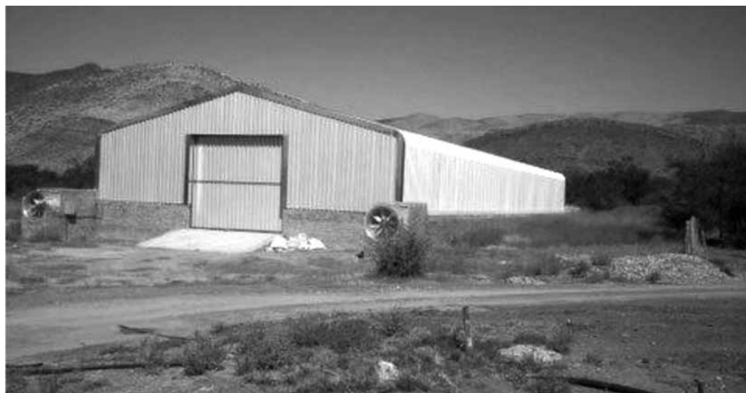
Figure 3.7: The shed for drying onion seed with extractor fans
