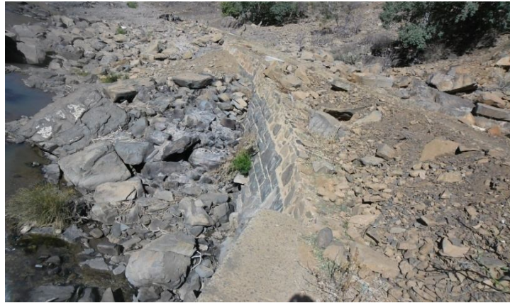
Plate 8: Concrete Pipe approximately 1.4 km long protected by a Retaining Wall
