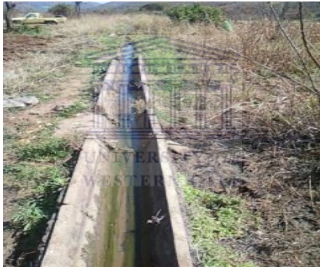
Plate 11: Infield Distribution Canal.
